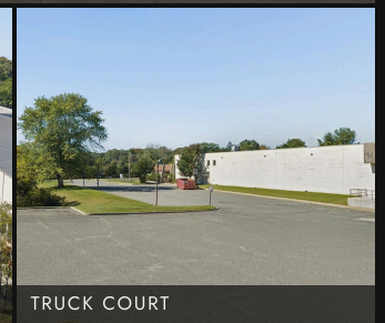
REAR PARKING AND TRUCK CO...
