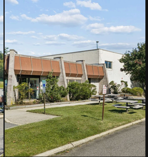
OFFICE ENTRY AND LANDSCAPED WALK
